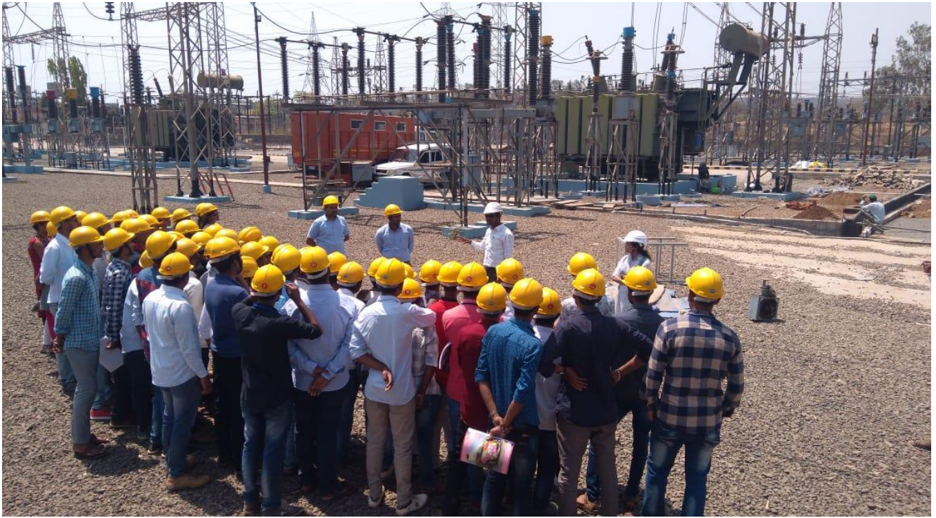
Substation 110kv/33kv Explanation by Mr. Bhushan Varke & Mr.Nitin K. Dake sir.
